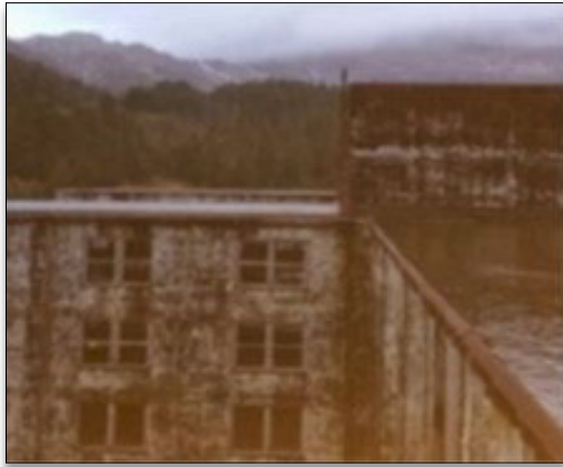
Buckner Building, Whittier
