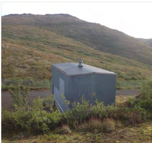
The Missile Assembly Building stabilization work is completed.
