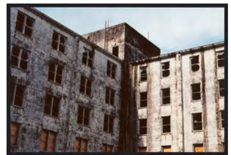
Buckner Building, Whittier
