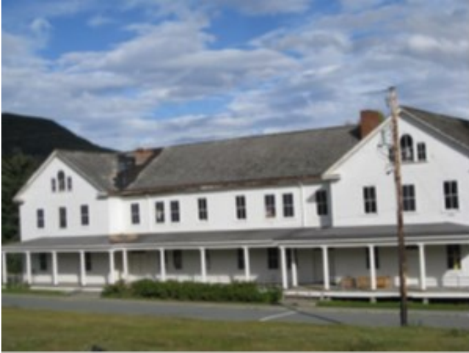
Barracks Building, Fort William H. Seward, Haines
