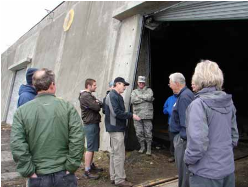
Site Summit veteran Greg Durocher explains the workings of the missile lifting system at Battery to VIPs and contractors who attended a FONSS tour in June 2011. The missile bunkers and other buildings at the upper and lower portions of Site Summit will be featured in the Aug. 8 VIP tour and the Sept. 8 public tour. (Photo by Doris Thomas)
