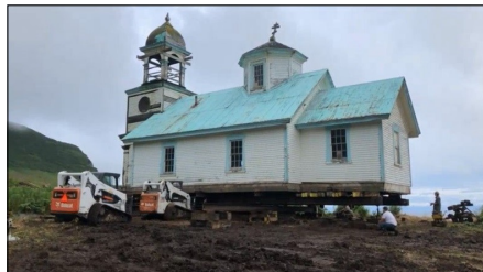
Two small bobcats begin the move away from the edge of the cliff. (Shina duVall photo)
