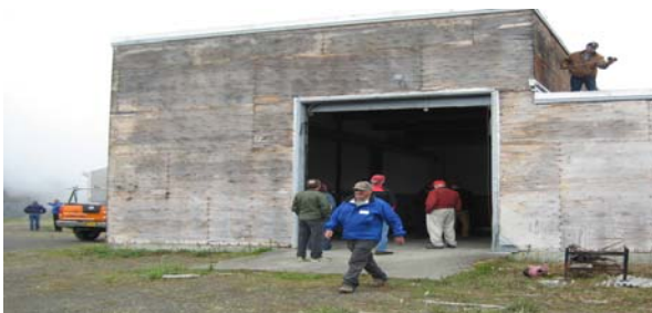
Pat Reilly of Rainproof Roofing takes measurements on the roof of the Launch Control Building. (Photo by Doris Thomas)
