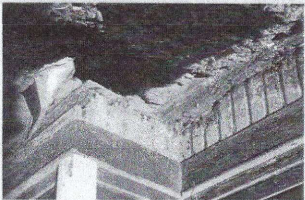
The photo above shows the Wasilla railroad depot; below is a detail showing the extent of dry rot on the exterior walls.
