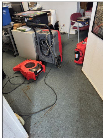
Fans were set up throughout the basement to dry out the basement. They ran for over a week.
